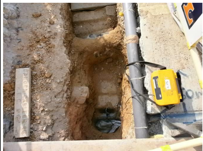
Figure 11 Locator setup at 275kv electric cable
