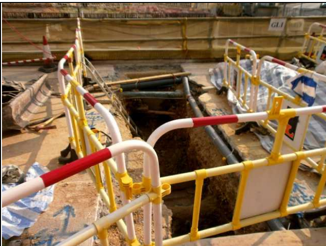
Figure 7 Trial pit T/P A
