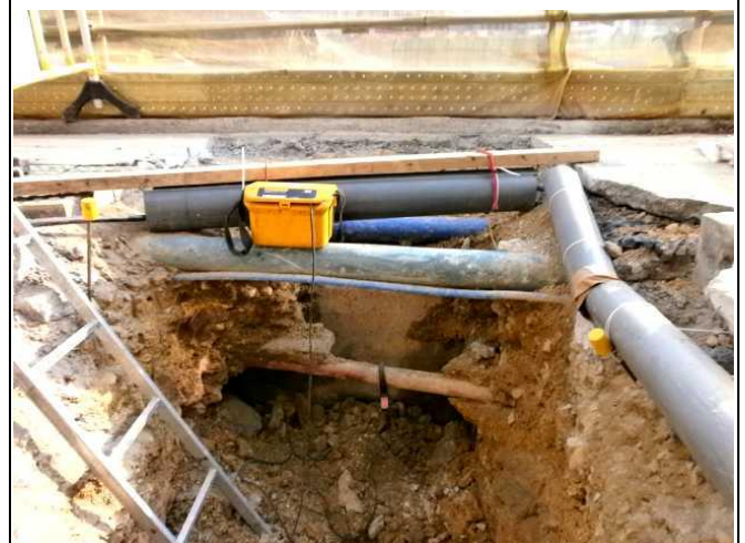
Figure 12 Locator setup at 11kv electric cable
