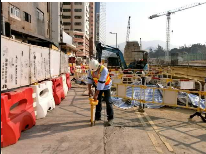
Figure 15 Locating in progress
